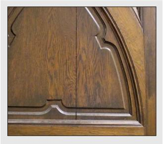
The panel of this old church door has a split. The door is located next to a radiator, exposing the wood to extremely low humidity levels, which more than likely caused the panel to contract and eventually split.
